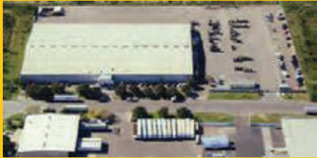
PROLAMSA LAREDO Laredo, TX Services offered: Cut-to-length, laser cutting, forming, bending, welding, deburring, reaming and chamfering.
