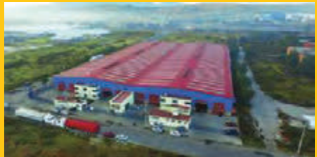
TEPEJI PLANT Tepeji del Río, Mexico
