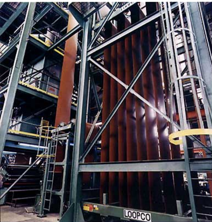
Paint line at Prolamsa's Monterrey plant.
